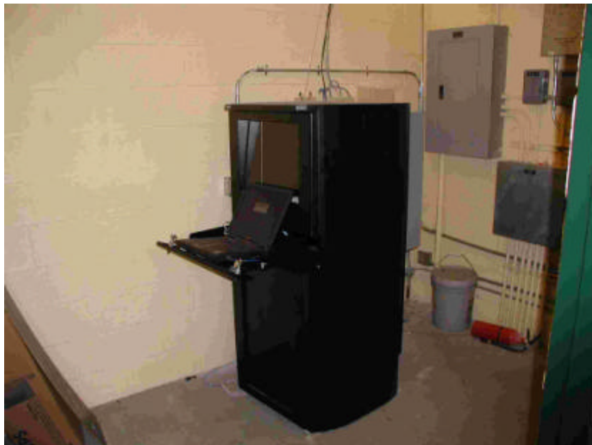
Figure 22 Rail CrossingGuard Server Installed at Cypress Creek Station
