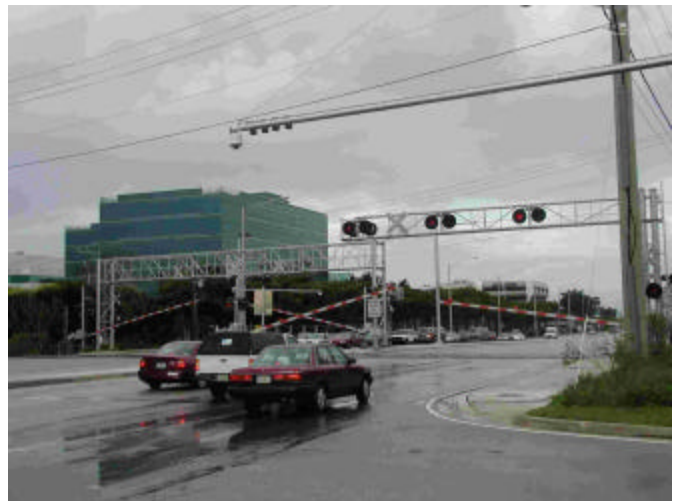
Figure 20 Signal Cameras Installed at Cypress Creek Road
