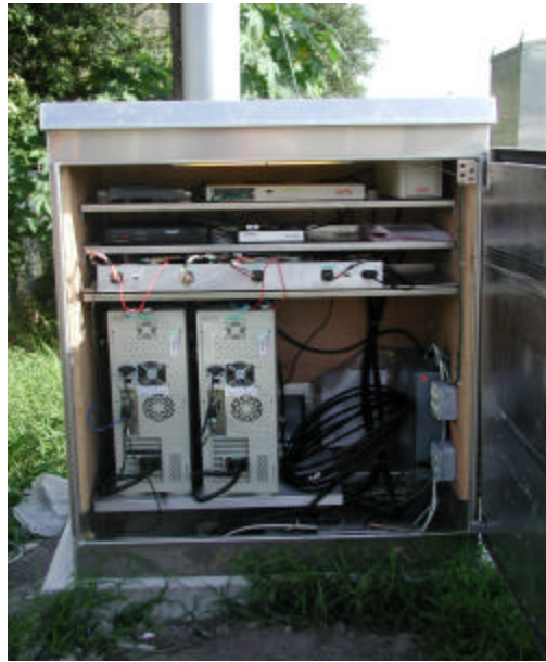
Figure 18 Rail CrossingGuard TrackSide Station (Image shows two TrackSide Stations in a controller cabinet.)
