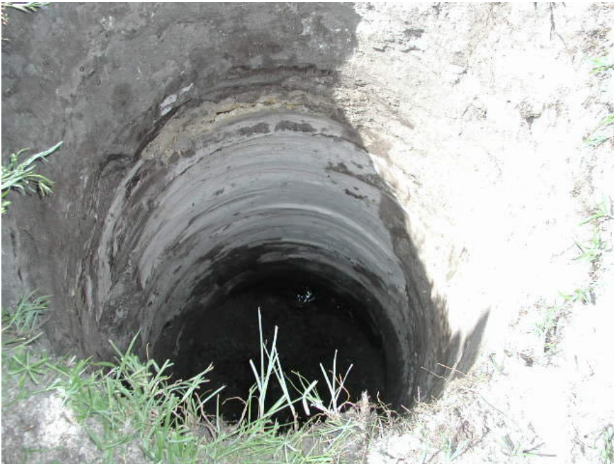
Figure 4 Close Up Looking Down Drilled Shaft for Camera Pole Foundation at Commercial Boulevard
