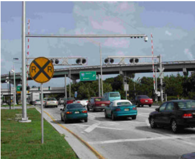
Figure 19 Signal Cameras Installed at Commercial Boulevard
