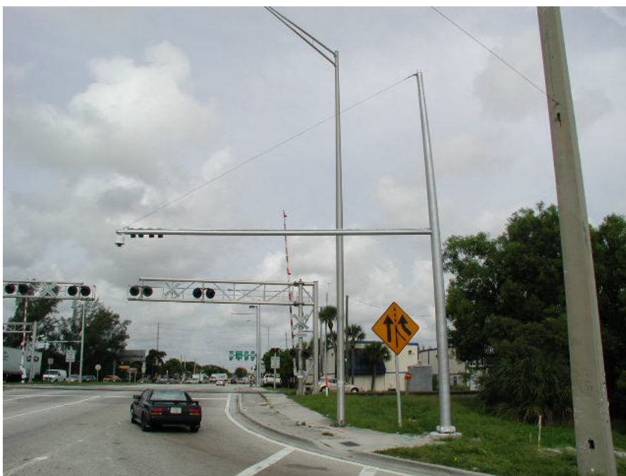
Figure 6 Fiberglass Pole Bending Under Load of Mastarm and Camera Copyright © 2002 Nestor Traffic Systems, Inc.
