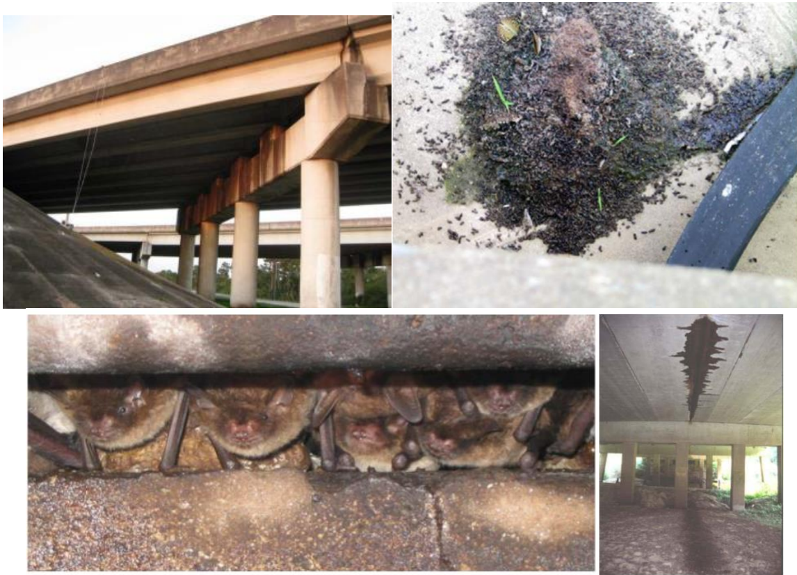
Top Left – Bridge staining. Top Right – Guano deposits visible from bridge deck. Bottom Left – Visible bats within an expansion joint. Bottom Right – Staining on underside of expansion joint and guano deposits on the ground.
