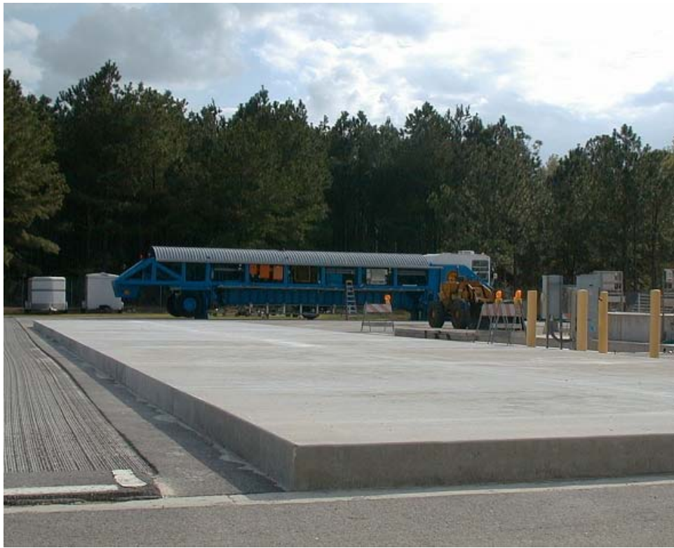
Figure 3. Finished concrete test track
