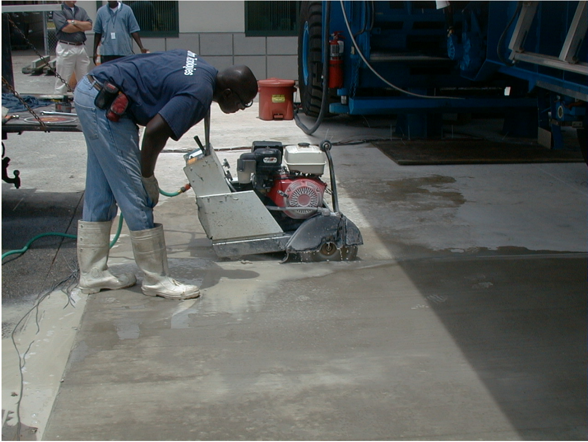
Figure 32. Making a 3-inch deep saw cut at the joint
