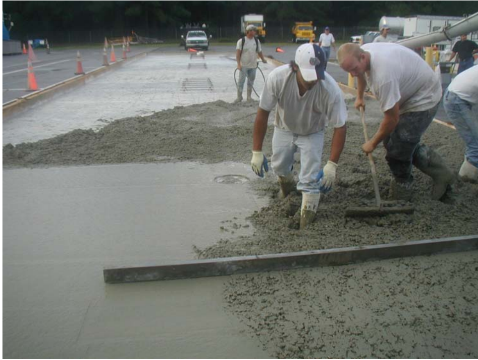
Figure 2. Placement of concrete on test track
