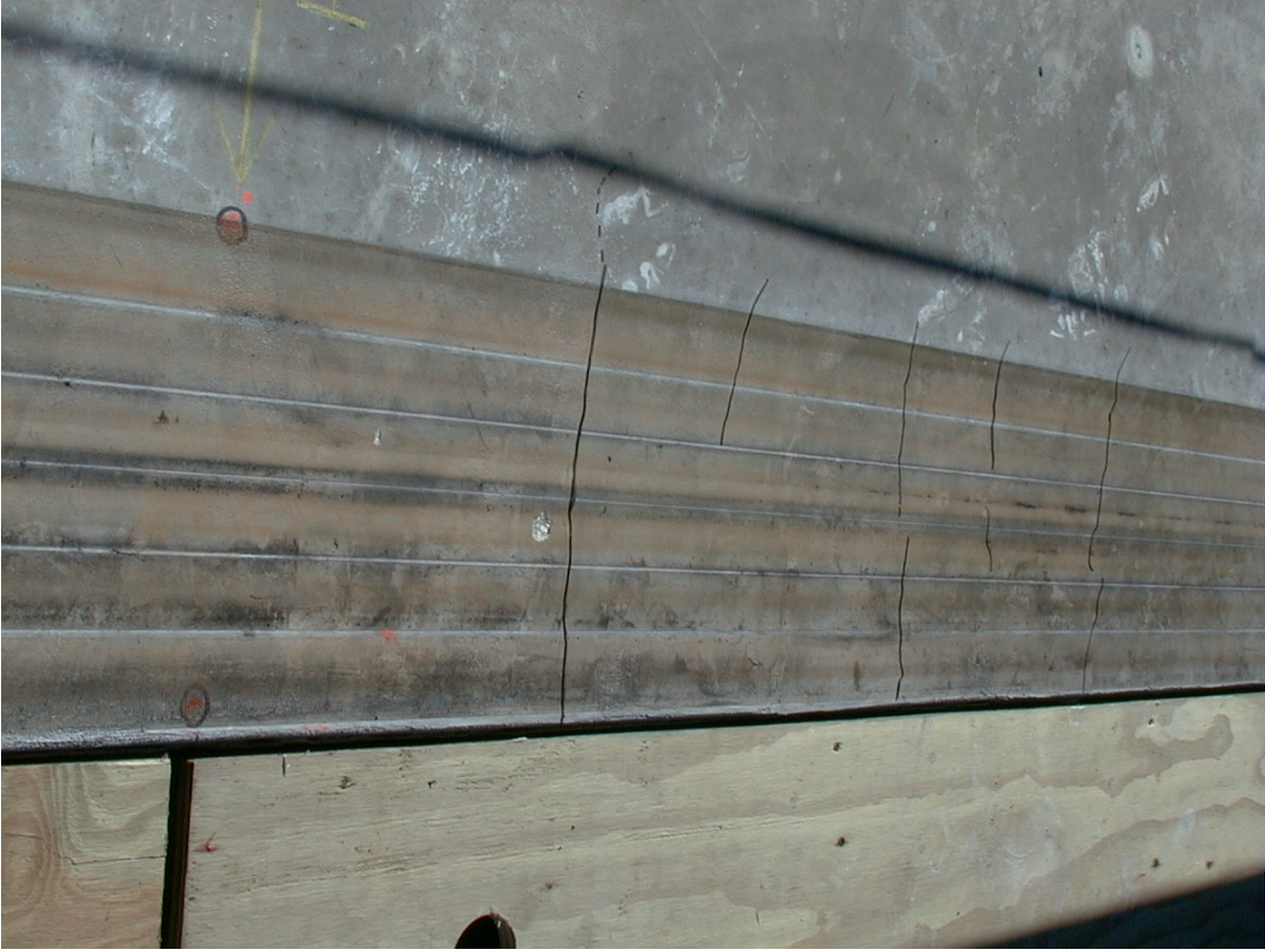
Figure 51. Cracks on Slab 2C at the end of HVS testing
