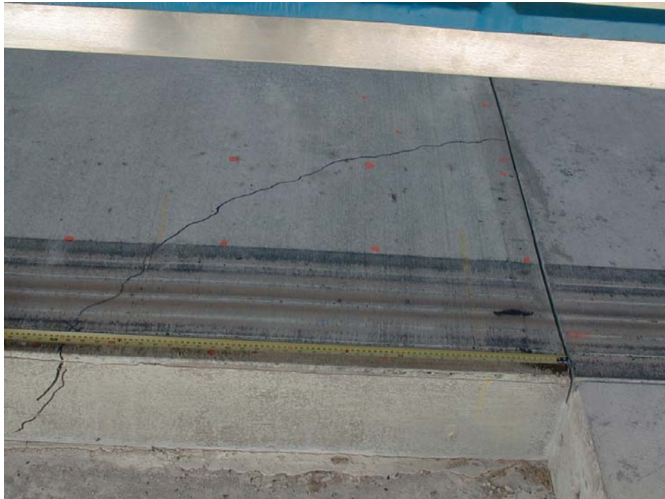
Figure 46. Corner crack at the southern end of Slab 1G
