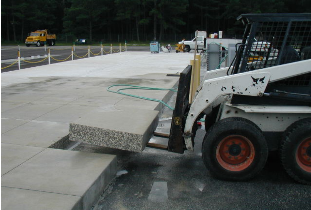
Figure 22. Removal of separated pieces using a lifter
