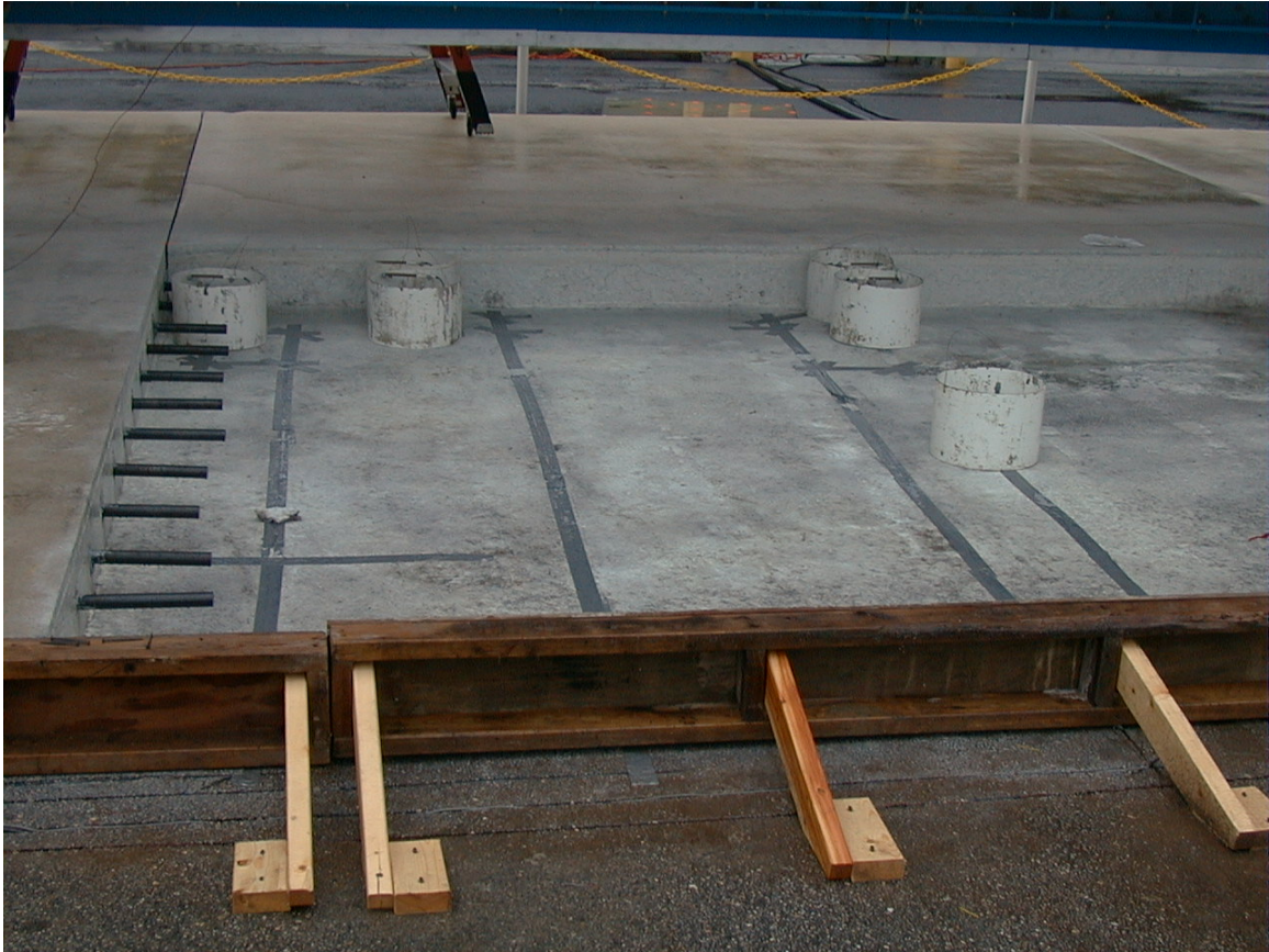
Figure 25. Dowel bars epoxied to an adjacent slab before placement of the test slab
