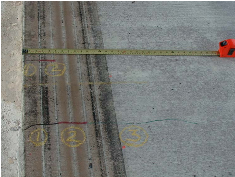
Figure 48. Crack propagation at the mid-edge of Slab 1G with additional loading
