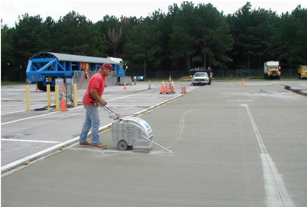
Figure 4. Making a 3-inch deep saw cut at the joint
