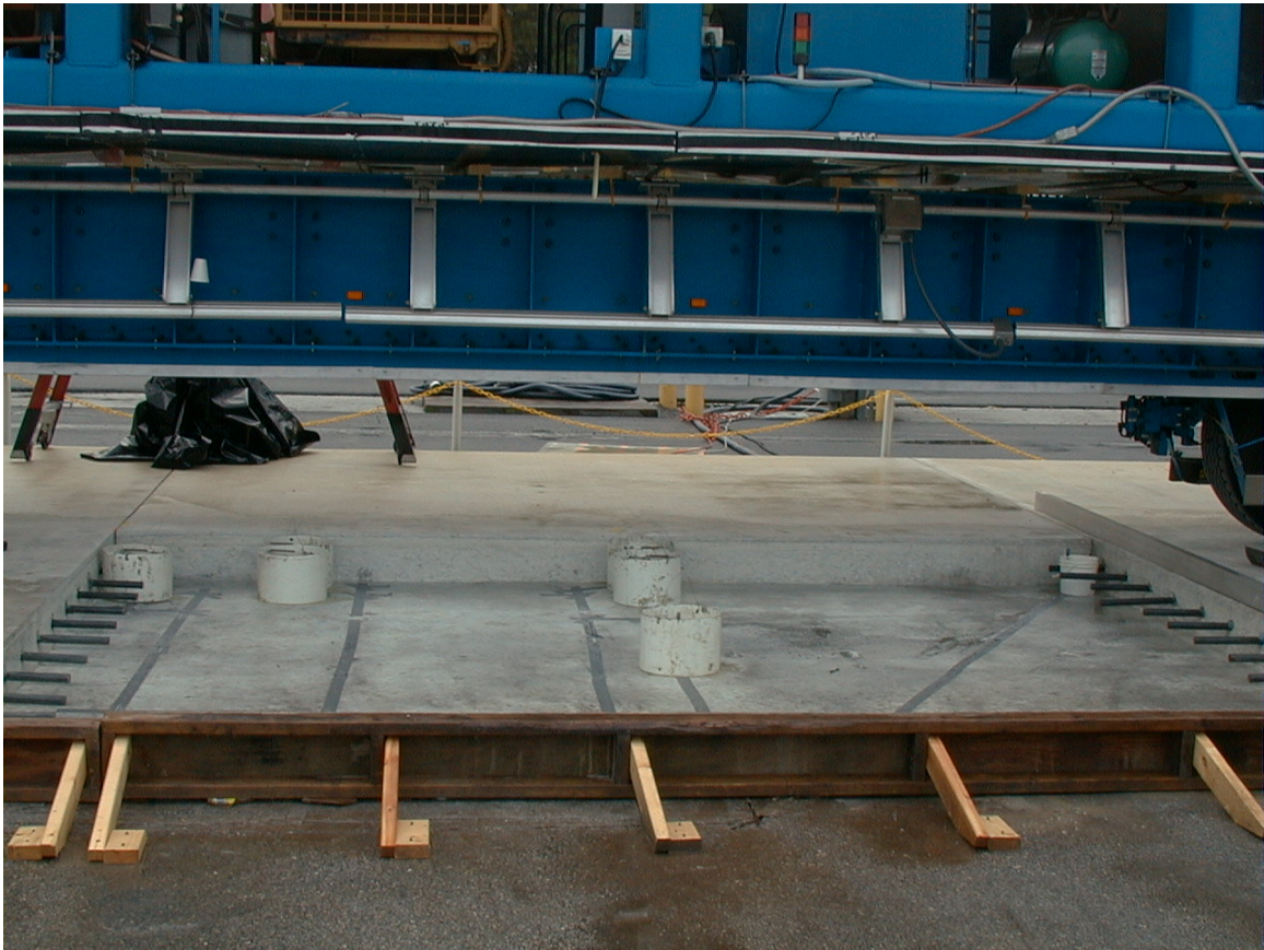
Figure 27. Formwork for the free edge of Test Slab 1C
