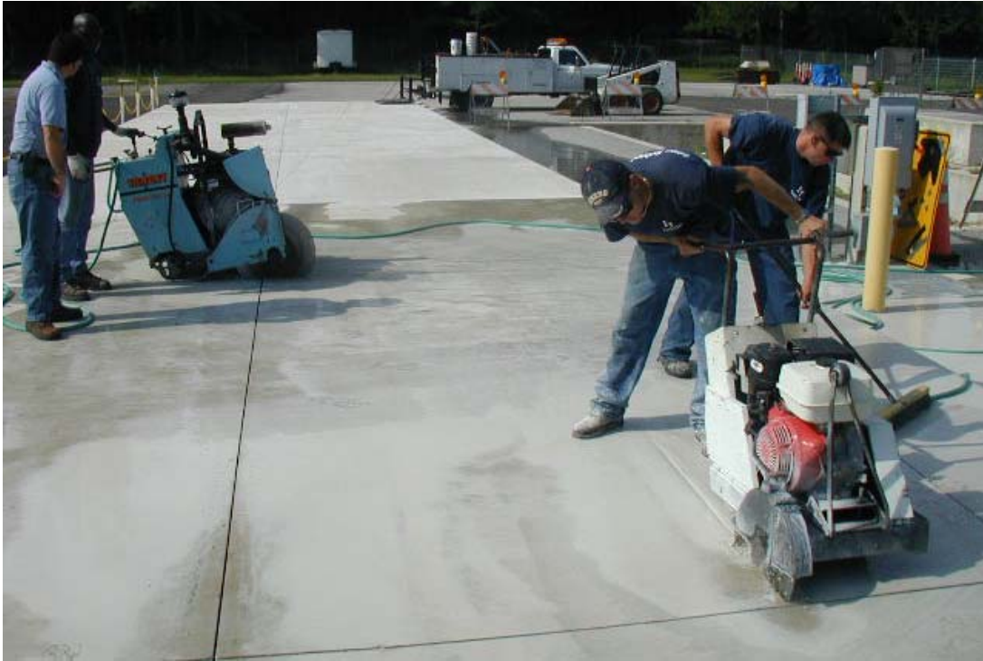
Figure 20. Cutting of a concrete slab (12 ft × 16 ft) into small pieces (3 ft × 4 ft)
