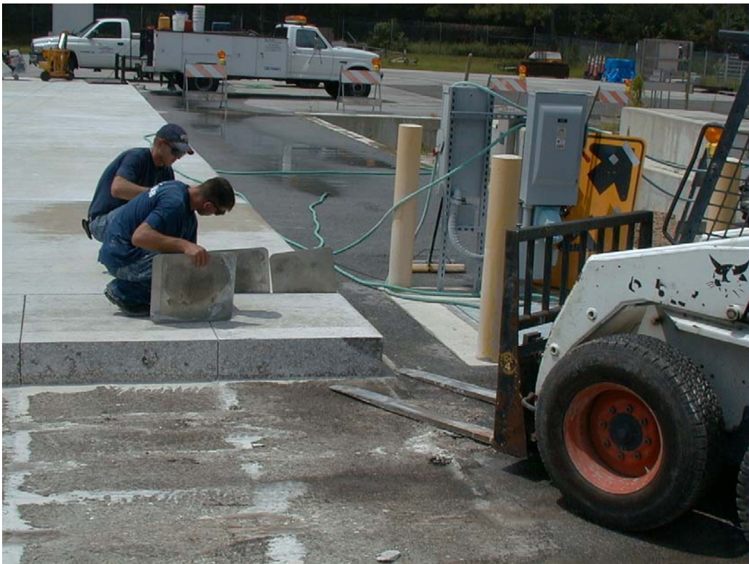
Figure 23. Removal of concrete pieces adjacent to the surrounding slabs
