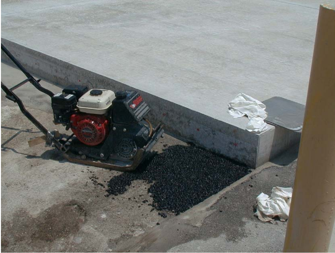
Figure 24. Correcting the damaged portion of the asphalt base
