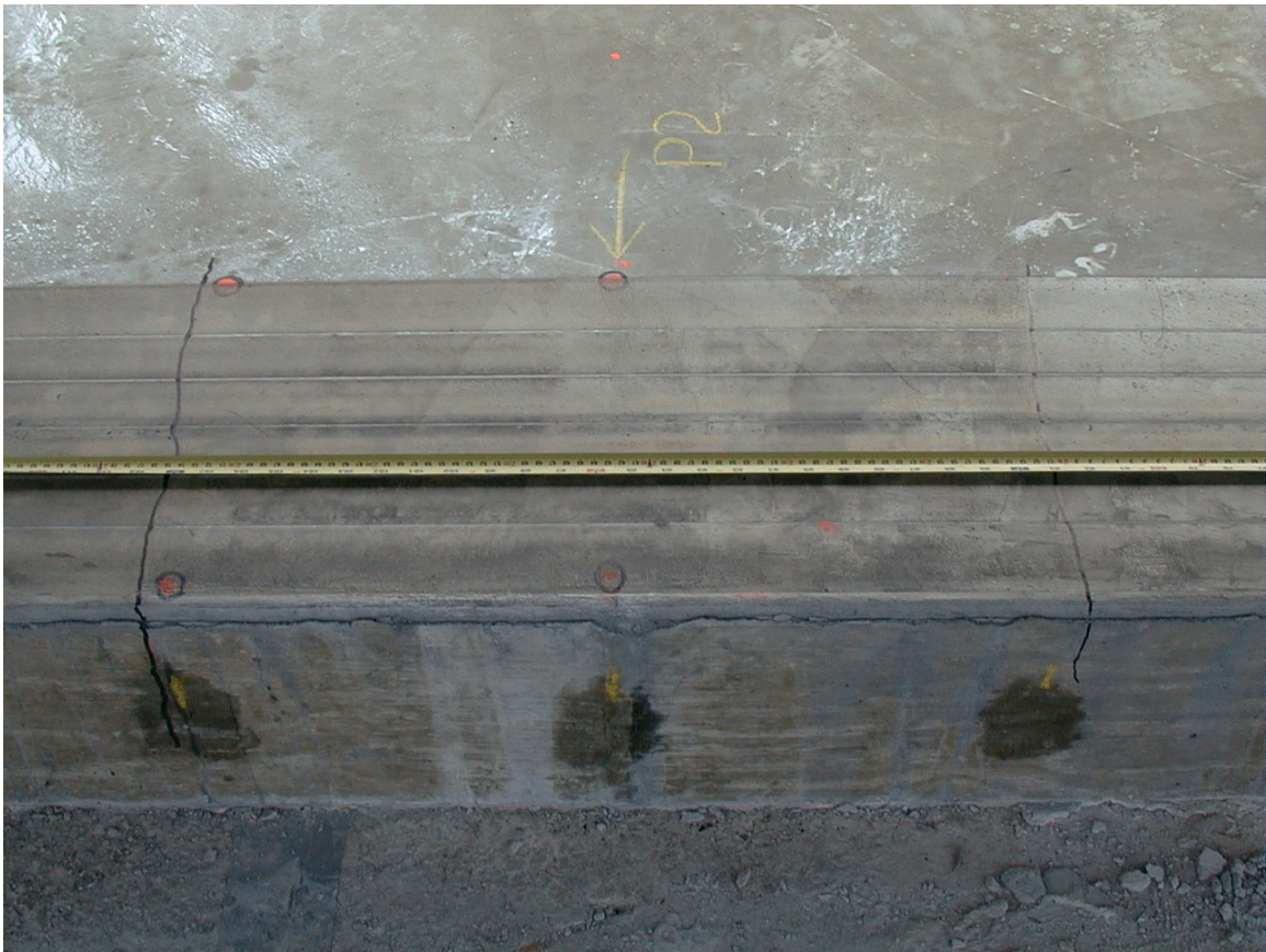
Figure 50. Transverse cracks at mid-edge of Slab 2C
