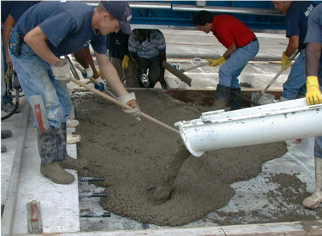
Figure 29. Placement of concrete for a test slab
