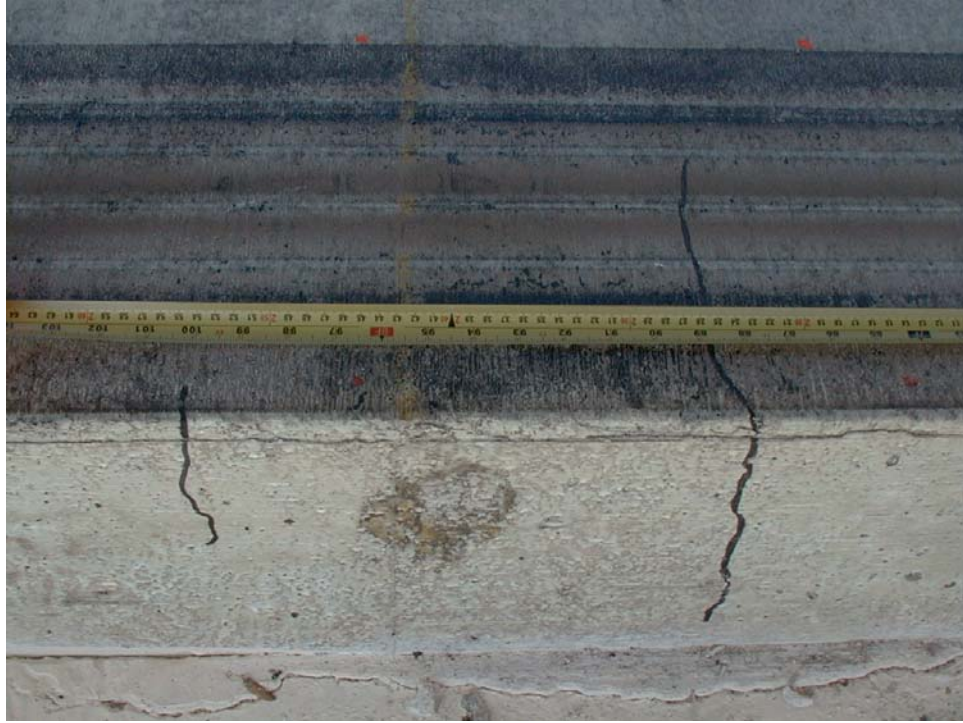
Figure 47. Transverse cracks at the mid-edge of Slab 1G
