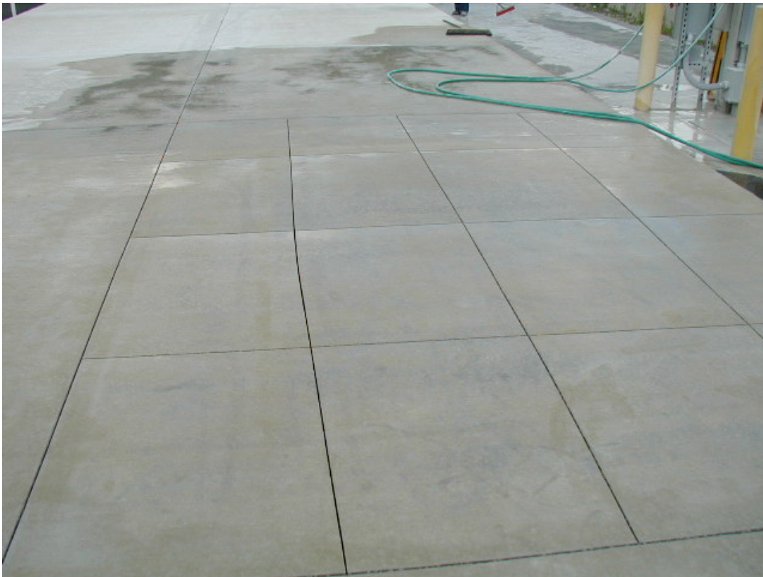
Figure 21. Separated concrete pieces after cutting with diamond bladed saw
