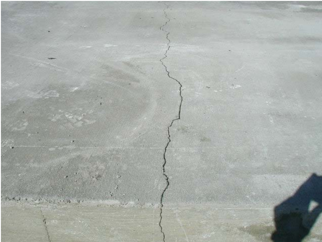
Figure 53. Transverse crack on Slab 2E at the middle of the slab
