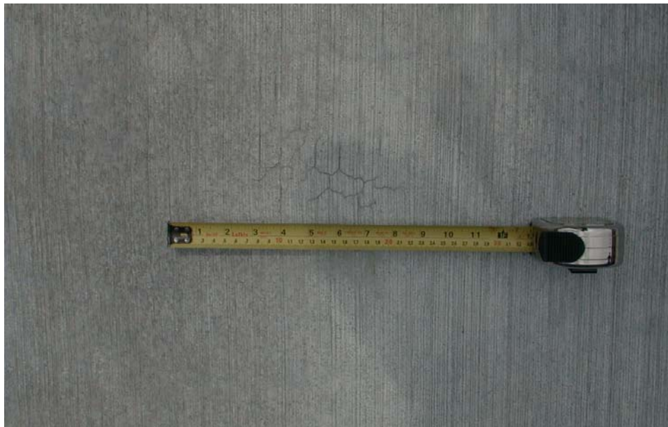
Figure 42. Shrinkage cracks on Test Slab 1C
