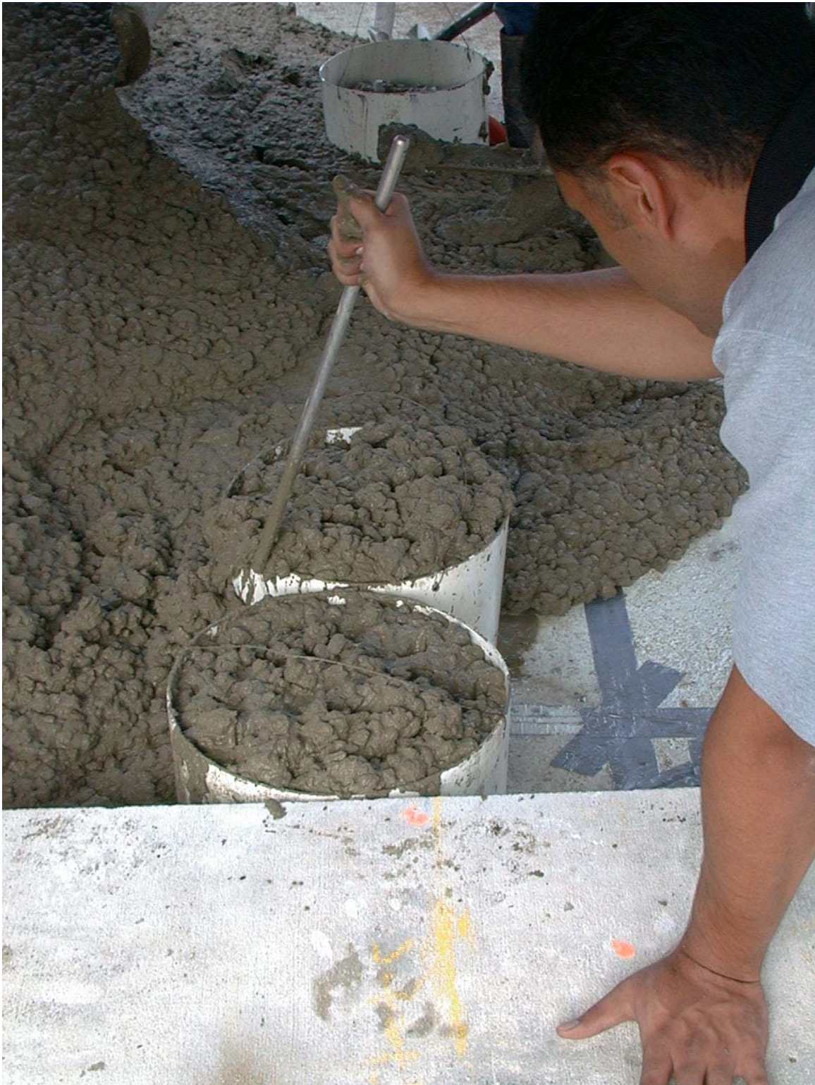
Figure 28. Placing concrete around strain gauges
