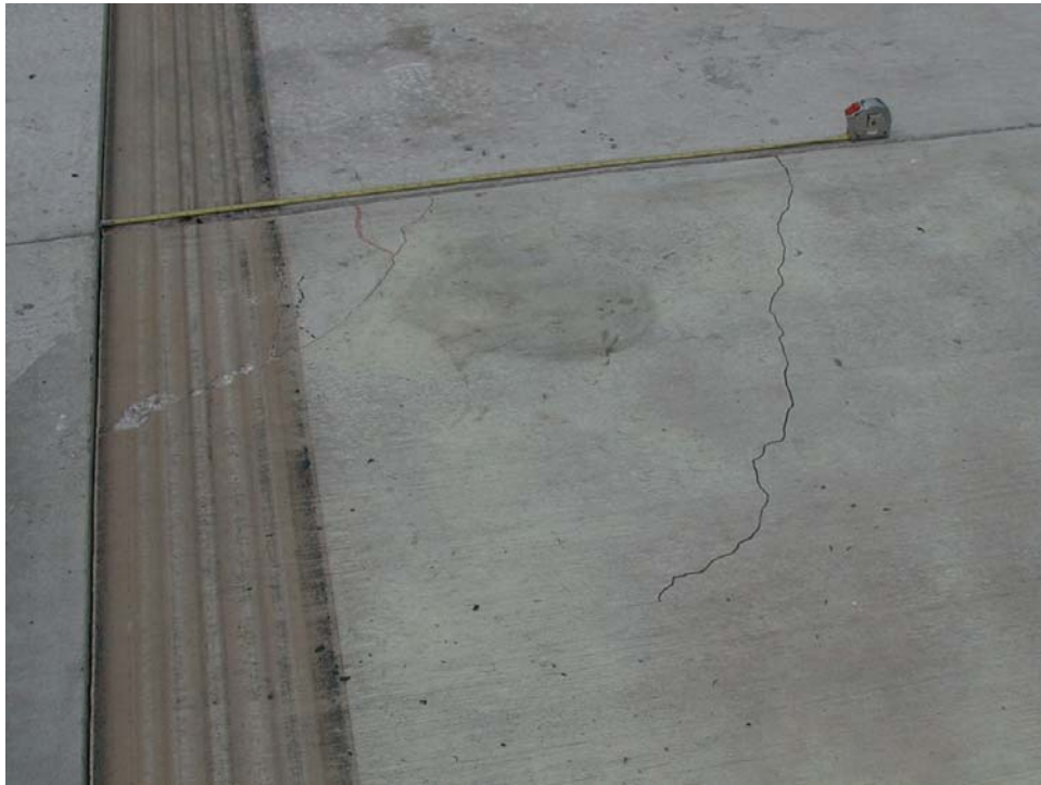
Figure 44. Cracked Slab 1C at the end of HVS testing
