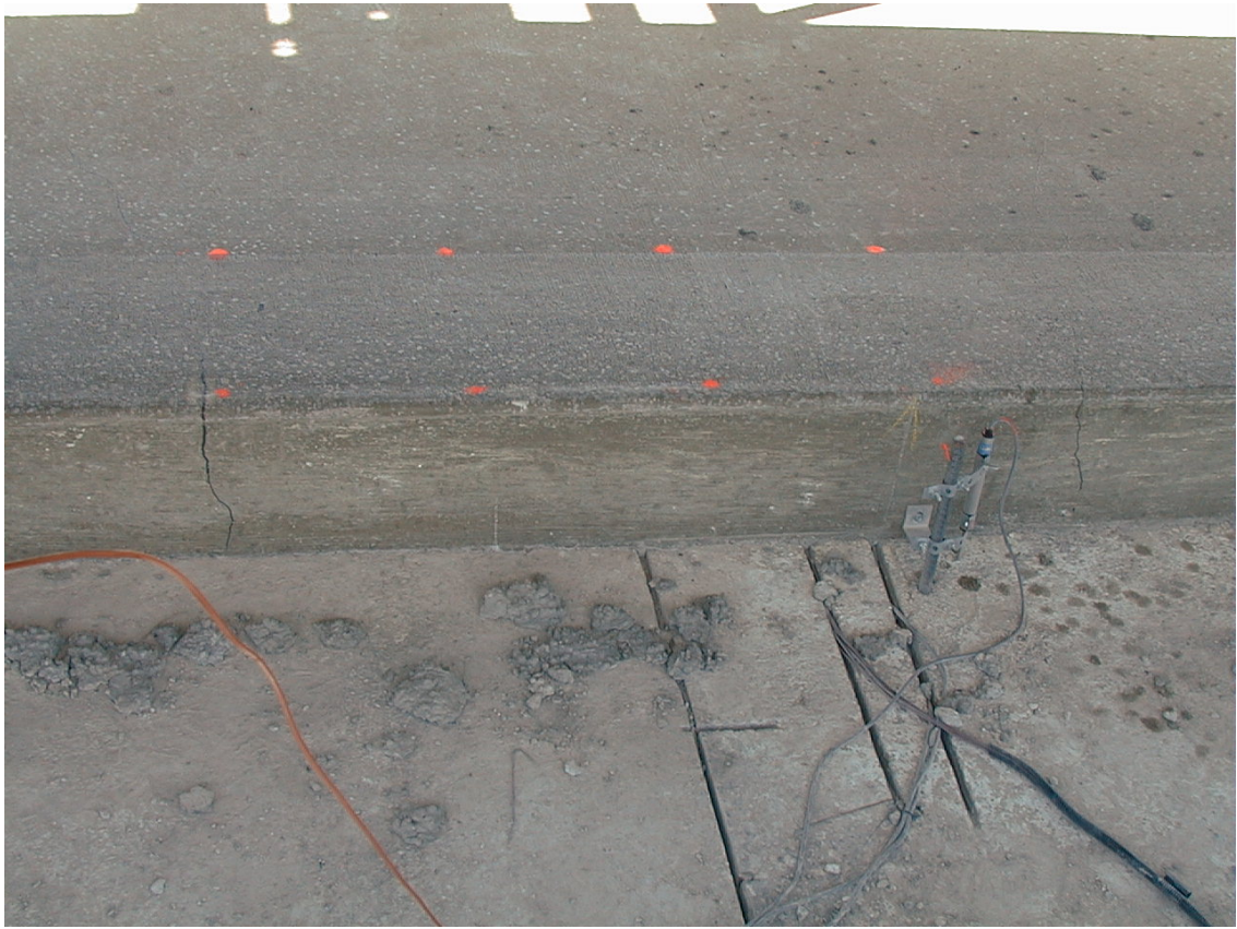
Figure 55. Transverse cracks on Slab 2G at the middle of the slab
