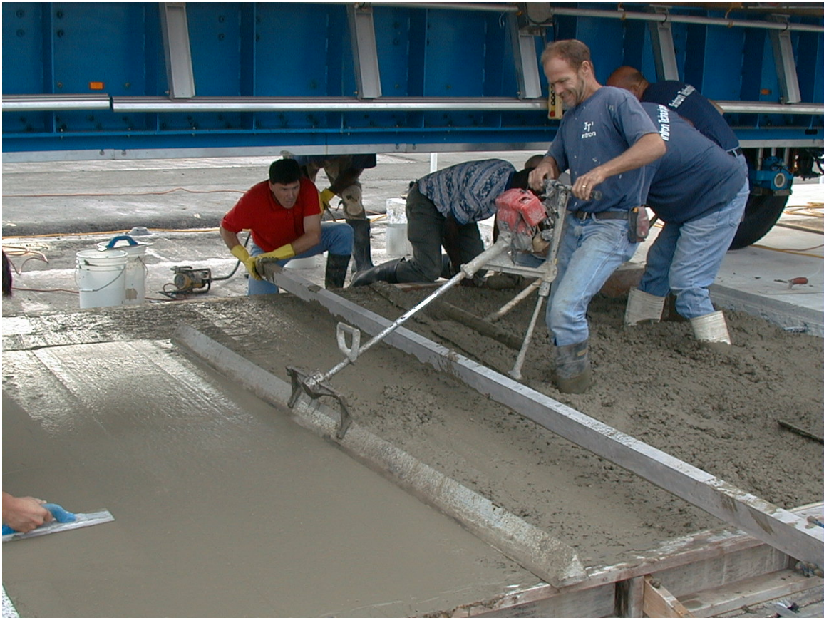
Figure 31. Leveling of concrete surface
