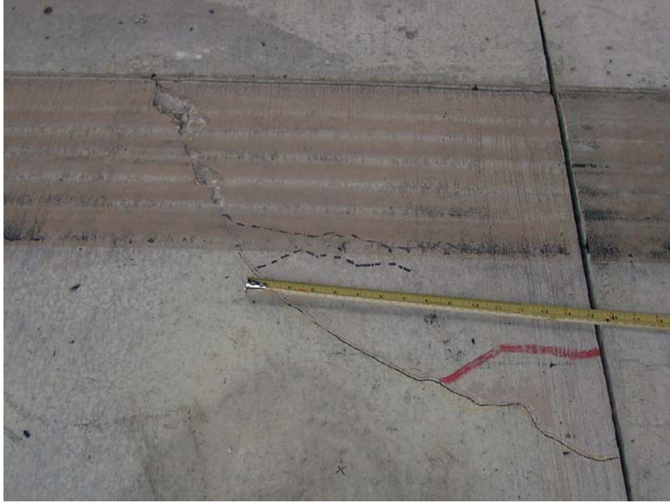
Figure 43. Corner crack on Slab 1C
