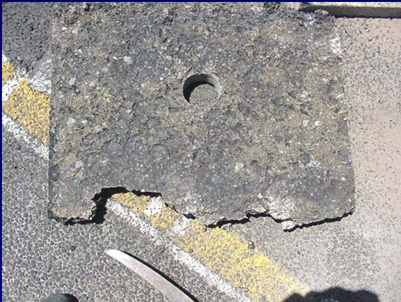
Underside of asphalt
