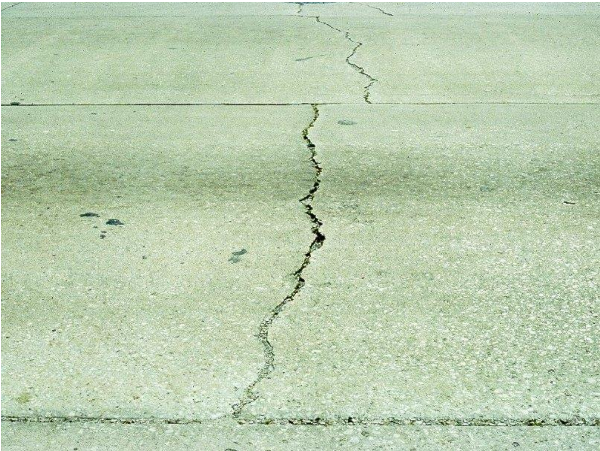
FIGURE 5. TRANSVERSE CRACKING
