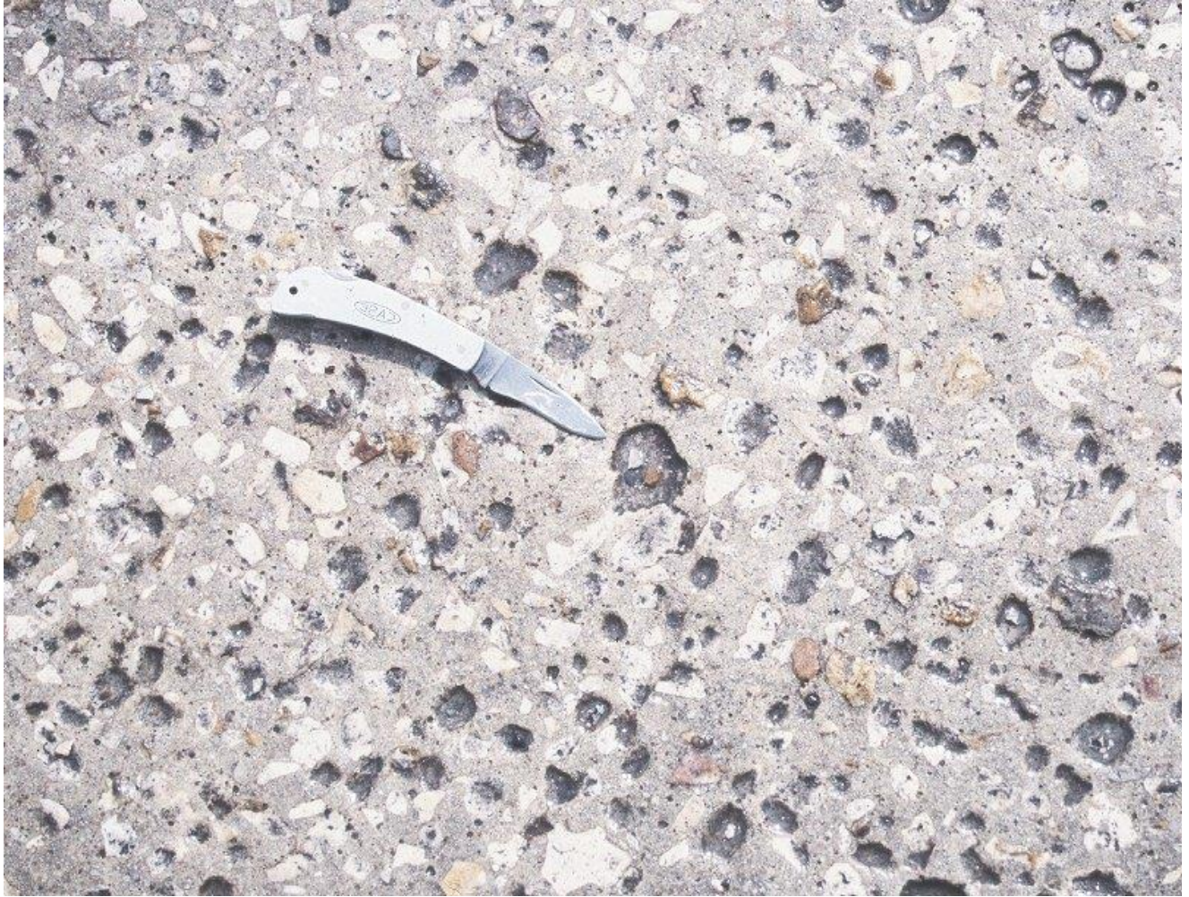
FIGURE 2. SURFACE DETERIORATION
