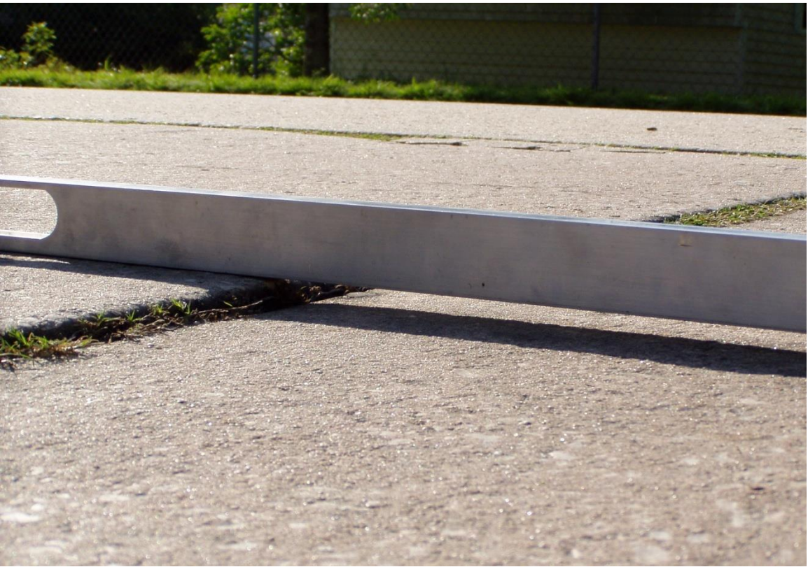
FIGURE 9. FAULTING
