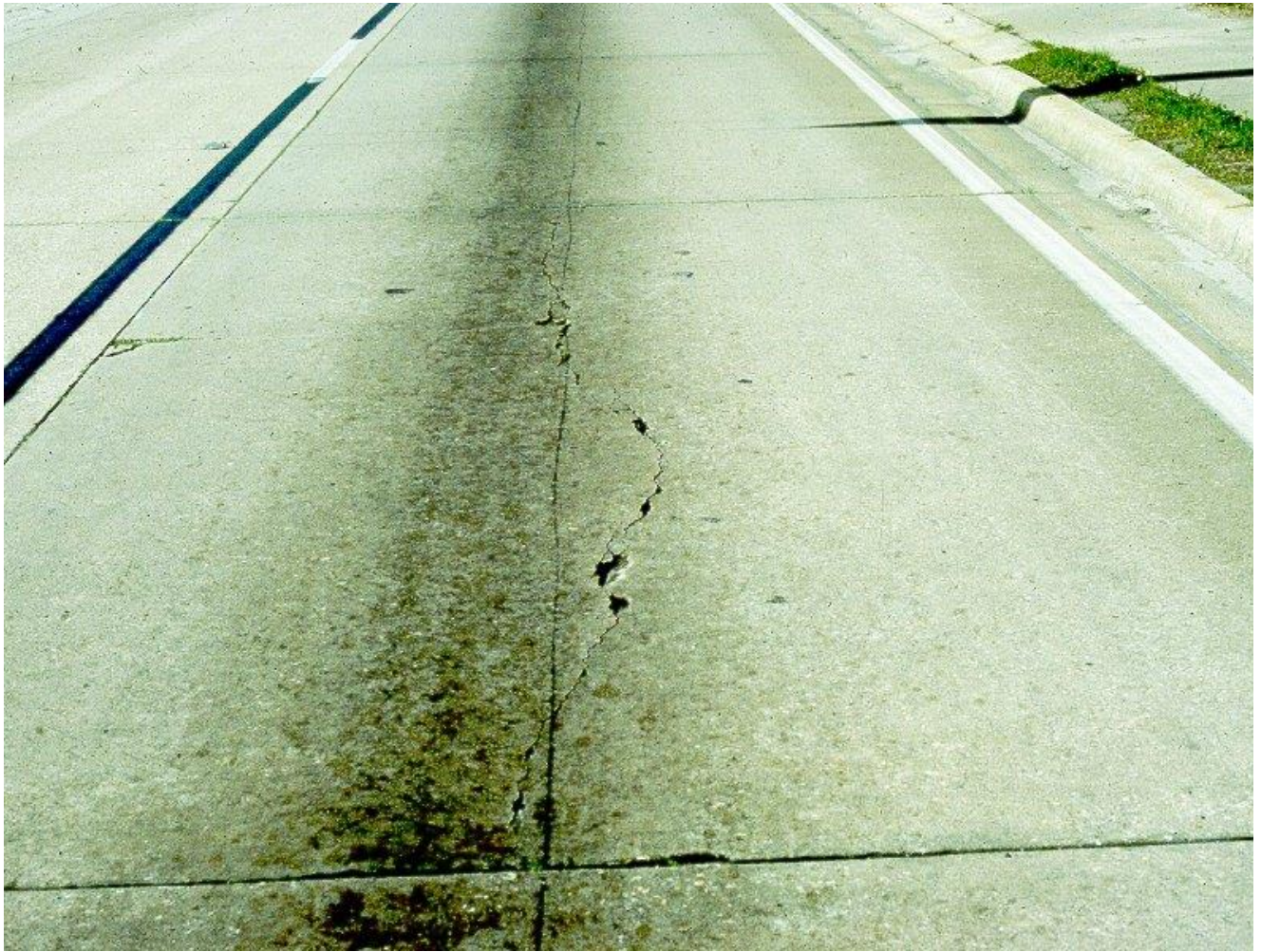
FIGURE 6. LONGITUDINAL CRACKING
