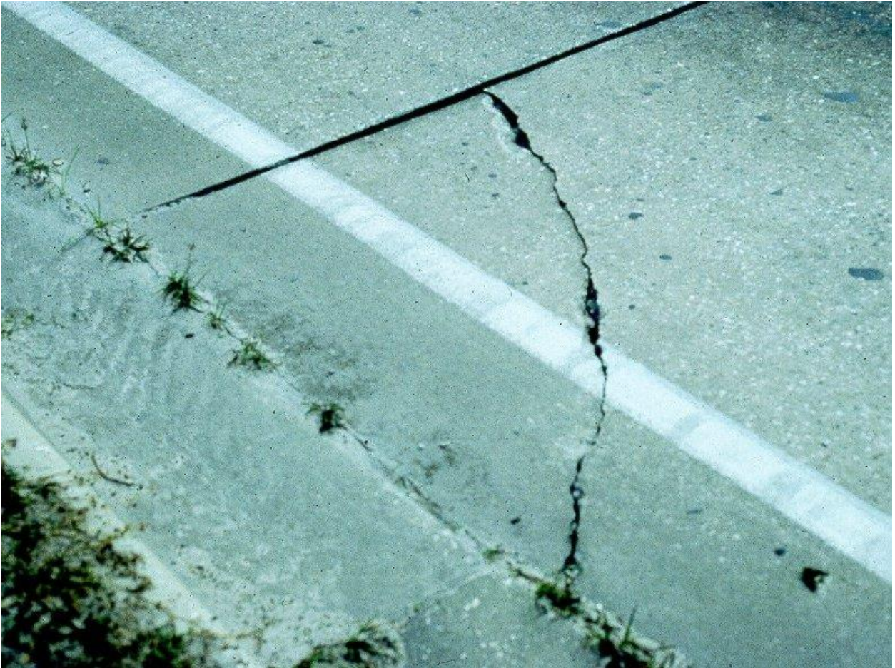
FIGURE 7. CORNER CRACKING
