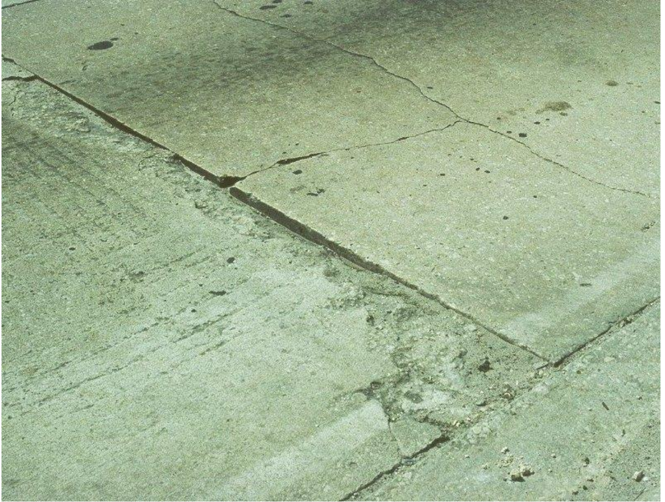
FIGURE 3. SPALLING
