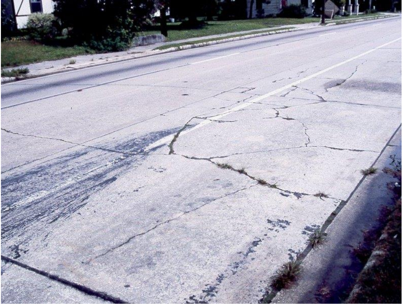
FIGURE 8. SHATTERED SLAB
