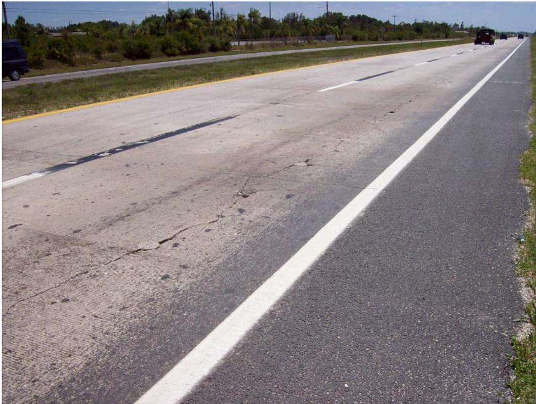
**FIGURE 12 Longitudinal cracking in section 2.**
