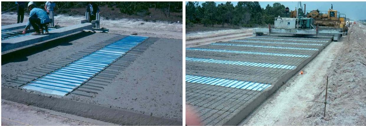
**FIGURE 6** Debonding material used for experimental joint concept (steel reinforcement shown).
