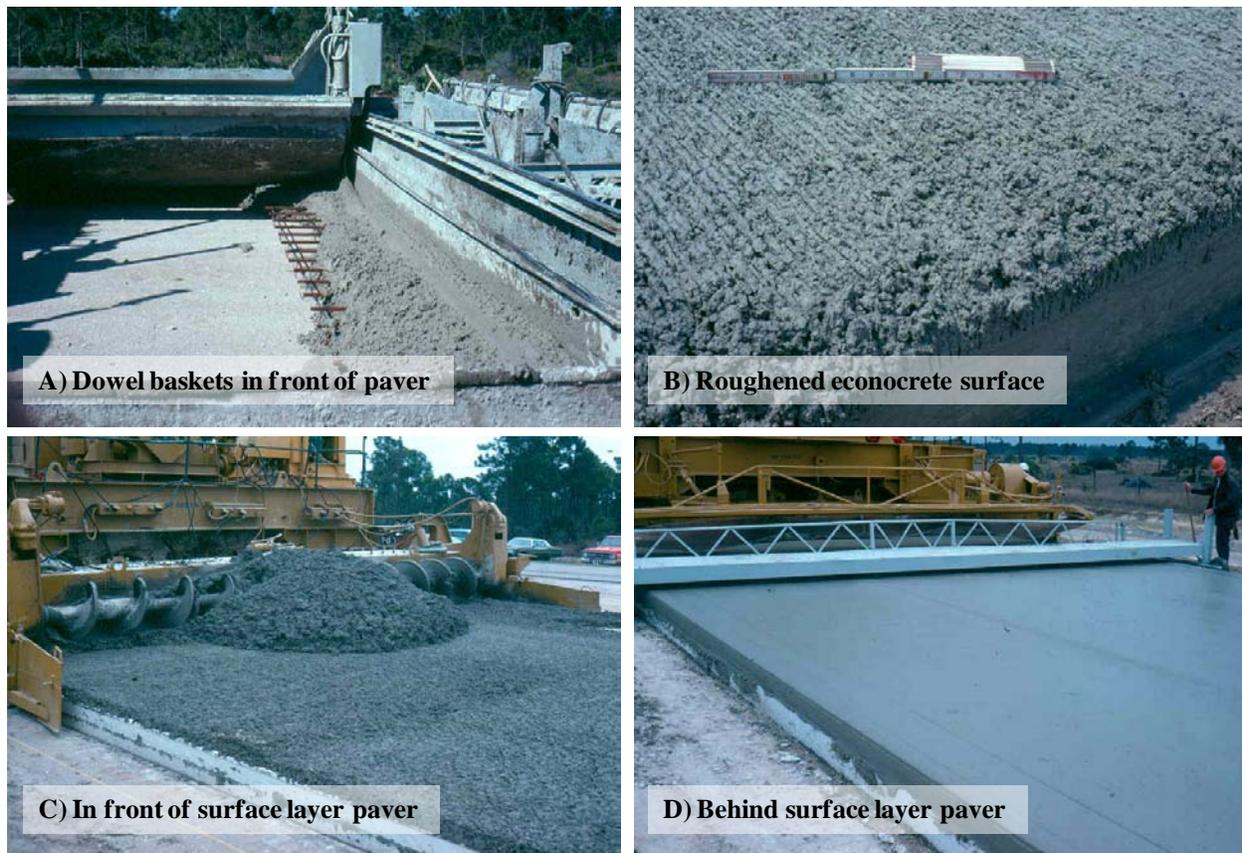
**FIGURE 3 Paving operation.**
