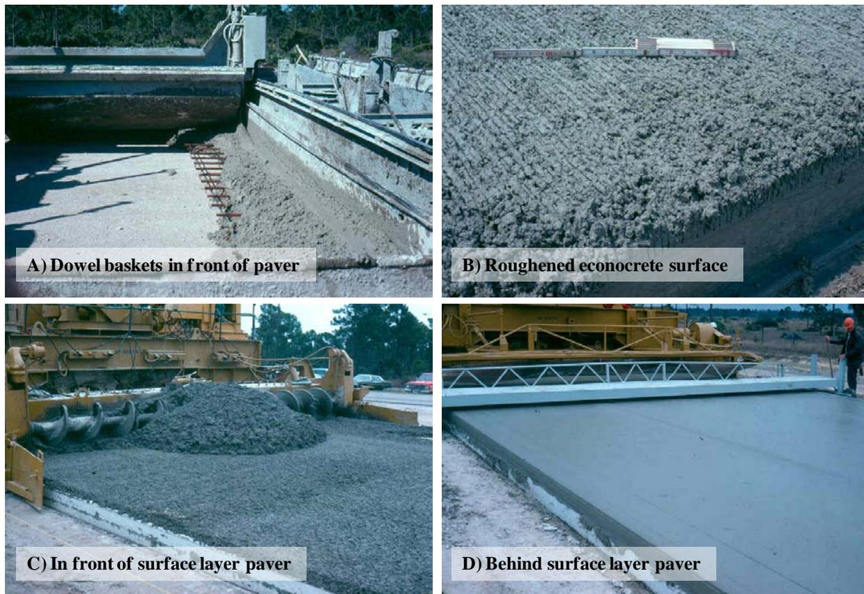
**FIGURE 3 Paving operation.**
