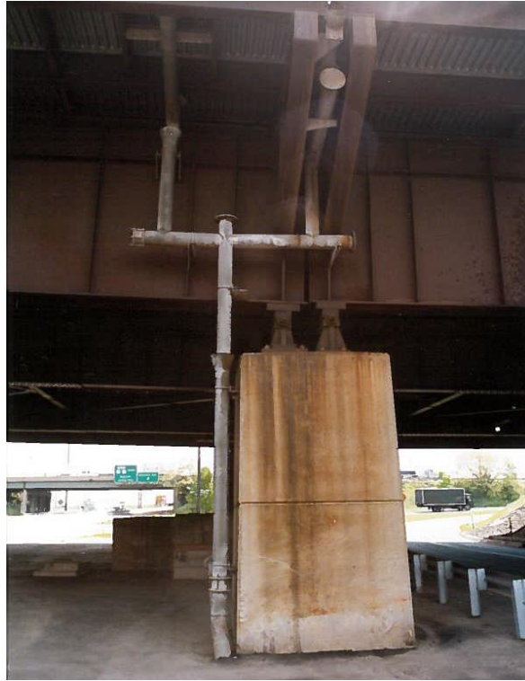
Figure 10.26 Closed Bridge Drainage with Orthogonal Piping Prone to Clogging (Courtesy of the New Jersey Turnpike Authority)
