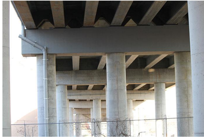
Figure 10.3 Photo of a Closed Bridge Drainage System – Fiberglass (Courtesy of FRPbridgedrainpipe.com)
