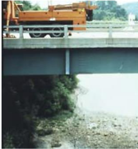
Figure 10.19 PVC Drain Extension Retrofit at Fascia
