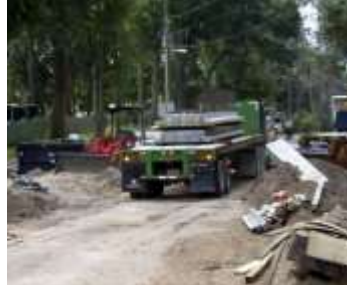
PRESTRESSED SLAB BEAMS (Gospel Island, FL) 25 kips x 2 = 50 kips Total 39 ft. beams
