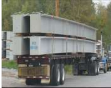
HYBRID COMPOSITE BEAMS (Union Street, ME) 9.0 kips x 4= 36 kips Total 70 ft. beams
