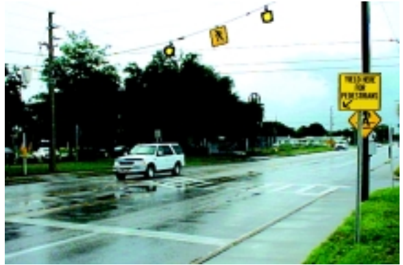
Special improvements made at the Menorah Center include the relocation of advance stop lines, a redesigned crosswalk, and the installation of overhead signals and prompting signs.
