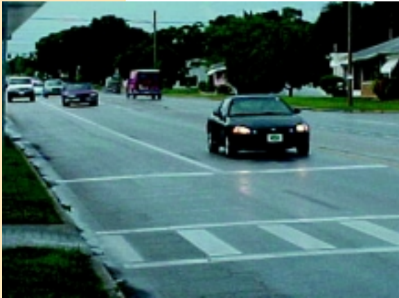
Advance stop lines were painted further away from the crosswalk to increase the distance between the motorist and the pedestrian.
